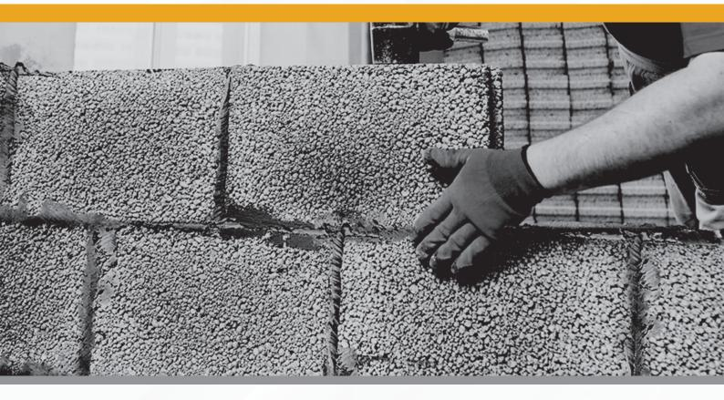
Block fix is a high Strength adhesive designed for swift and secure laying of AAC blocks with thin joints made from a blend of cement, graded sand and polymers making the surface water resistant with coatings as thin as 2mm.
